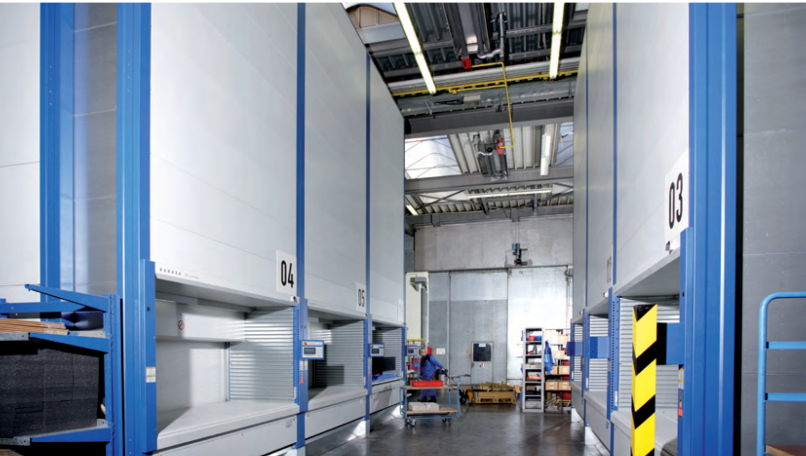
Computer controlled warehouse
